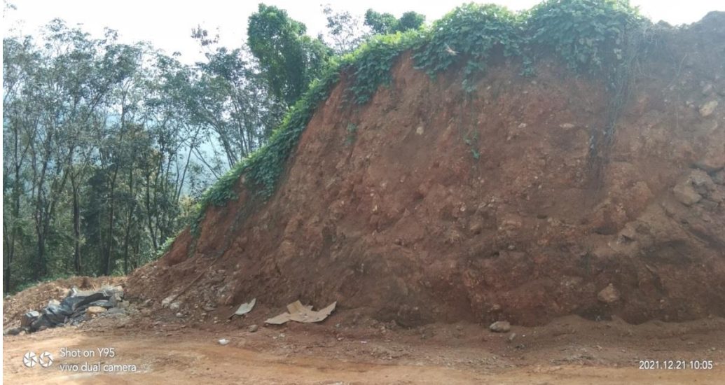
Figure 8: Photograph showing temporarily stored overburden dump
