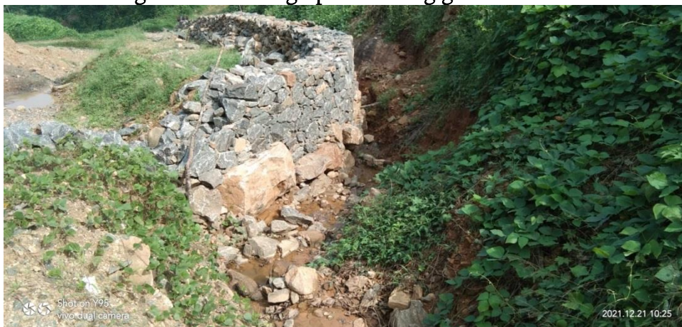
Figure I0 : Photographs showing garland drains
