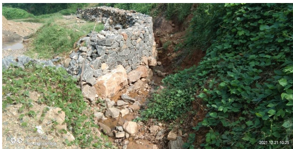
Figure 2 : Photographs showing garland drains
